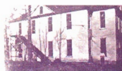
First School Building in Galax
